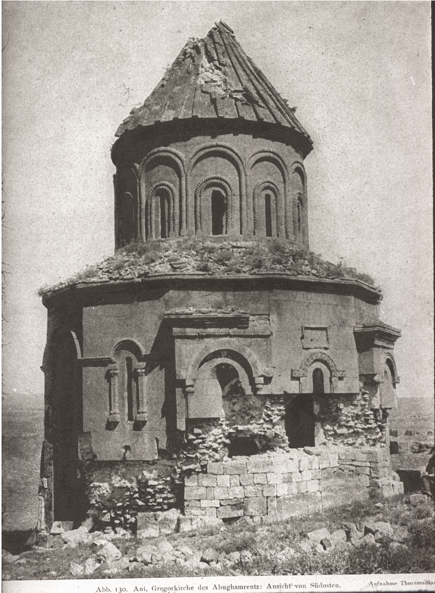
Figure 7.3. Toros Toramanyan. “Ani, Church of St. Gregory (Abghamrents). View from the Southeast.” Strzygowski, Die Baukunst , 1:127, fig. 130.
