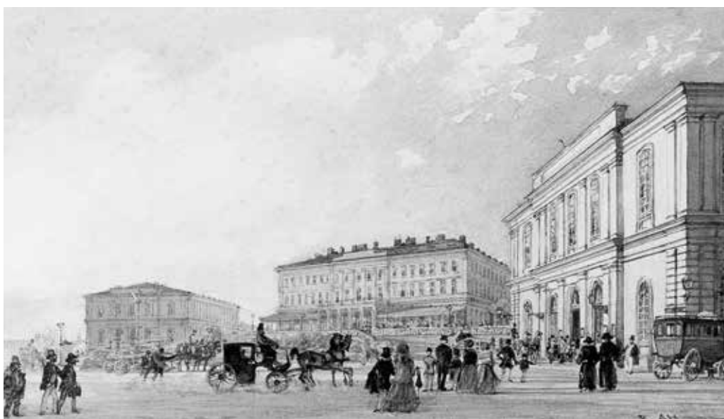
Fig. 7 Rudolf von Alt, The Gloggnitzer (right) and Brucker (left) railway stations near the Belvedere, on either side of an office building with a restaurant. Baedeker and Murray recommended this place to museum visitors for lunch. Watercolour, c. 1860. Vienna, ÖNB, Inv.no. D 16.735-B
