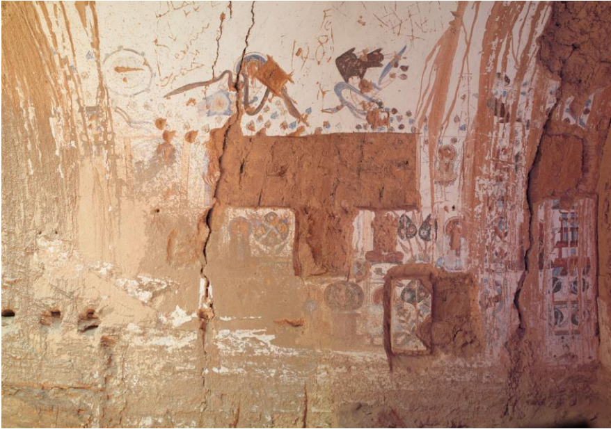
Fig. 16: Present state of the left wall of Toyok Cave 20. (Two pictures combined into one)
