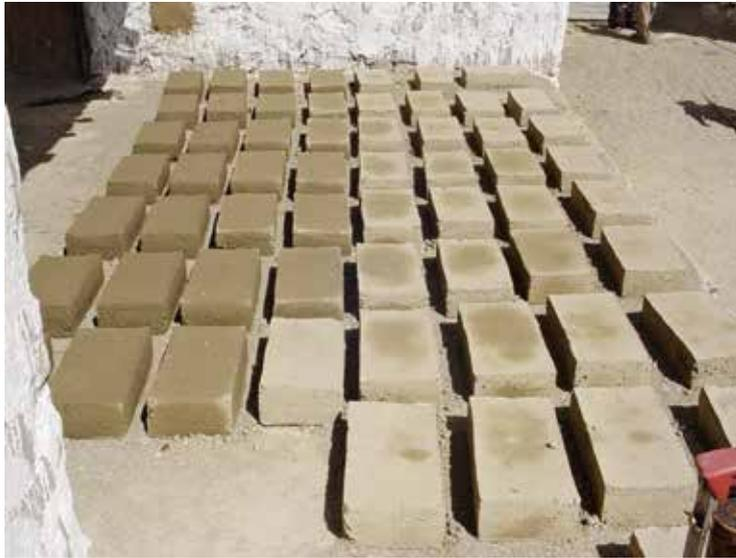
Fig. 56: Adobe mud bricks used for historical and conversation wall construction in the Western Himalayas.
