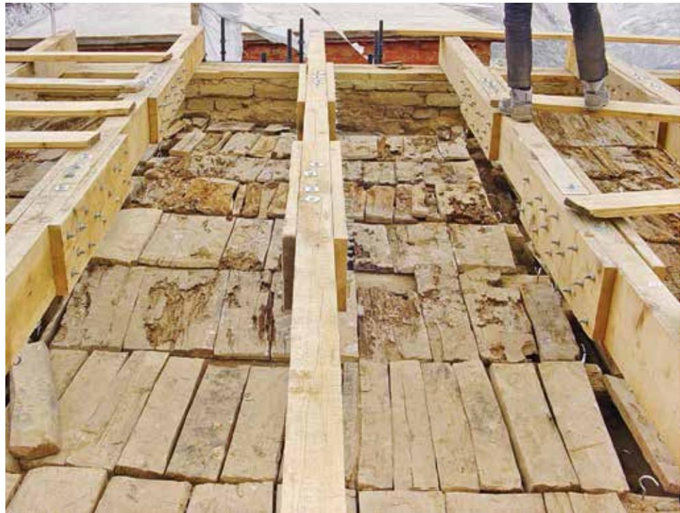
The historic ceilings and timber roof would be retained intact, conserved, consolidated and secured from the top but relieved of the unbearable weight. In addition, it would be protected by a new structural system comprising of nine beams and a layer of new ceiling planks laid on beams and new wall plates.
