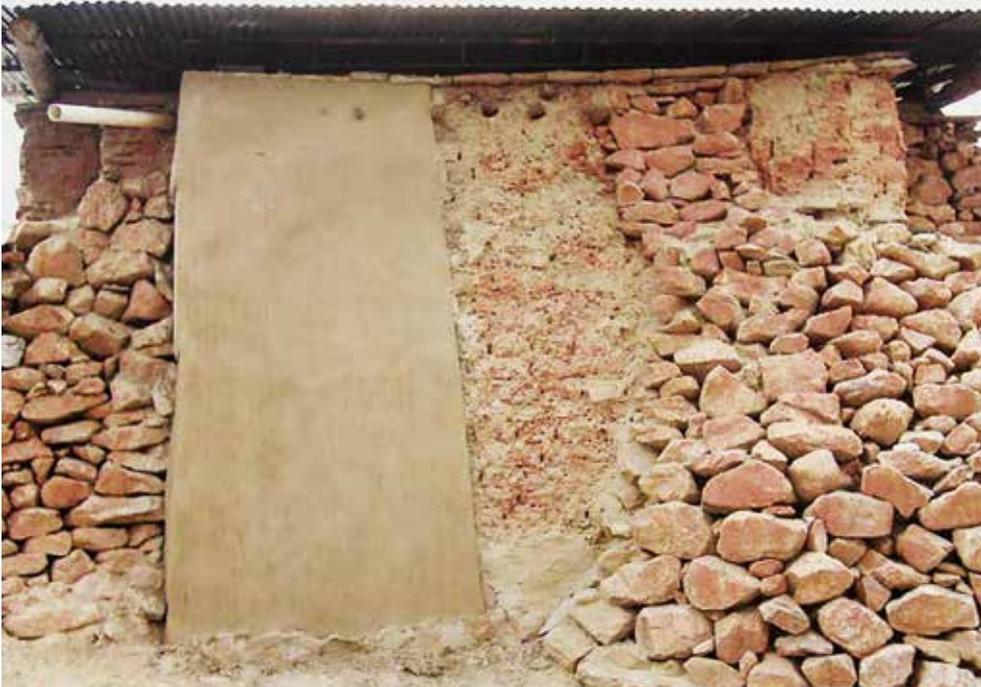
Fig. 191: Restored walls of Lhakhang Gongma with temporary roof cover during restoration.
