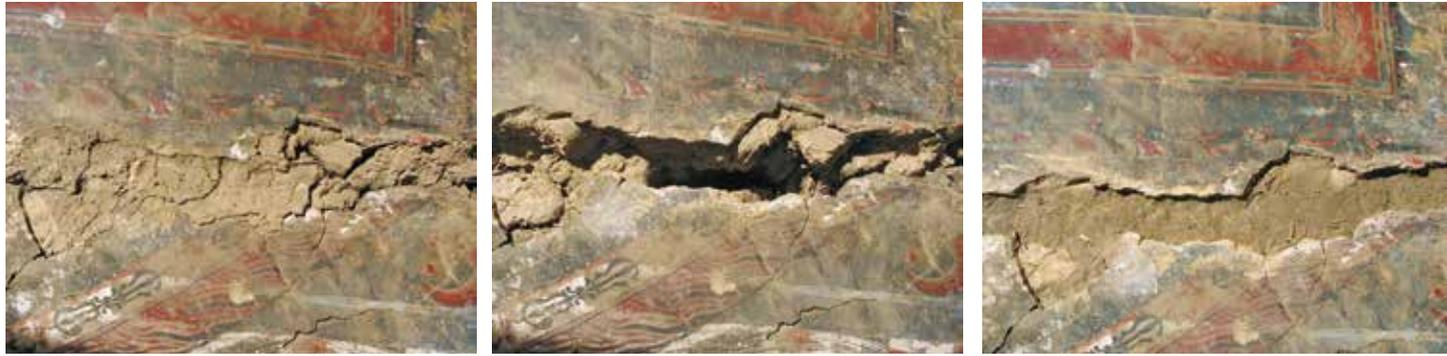
Fig. 236: Crack with old infill, Lhakhang Gongma.
