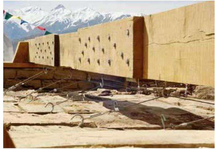
Fig. 189: Stainless steel cables provide a system of support to the original cracked beams.
