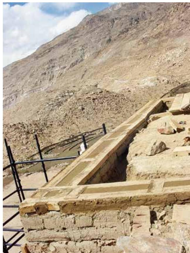
Fig. 186: Wall plates introduced at corners of parapet to strengthen structure at corners.
