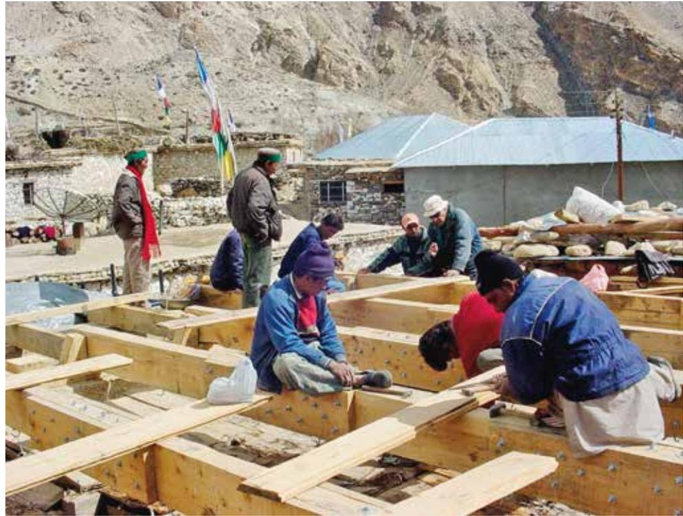
Fig. 184: New cedar beams are placed over historical roof.
