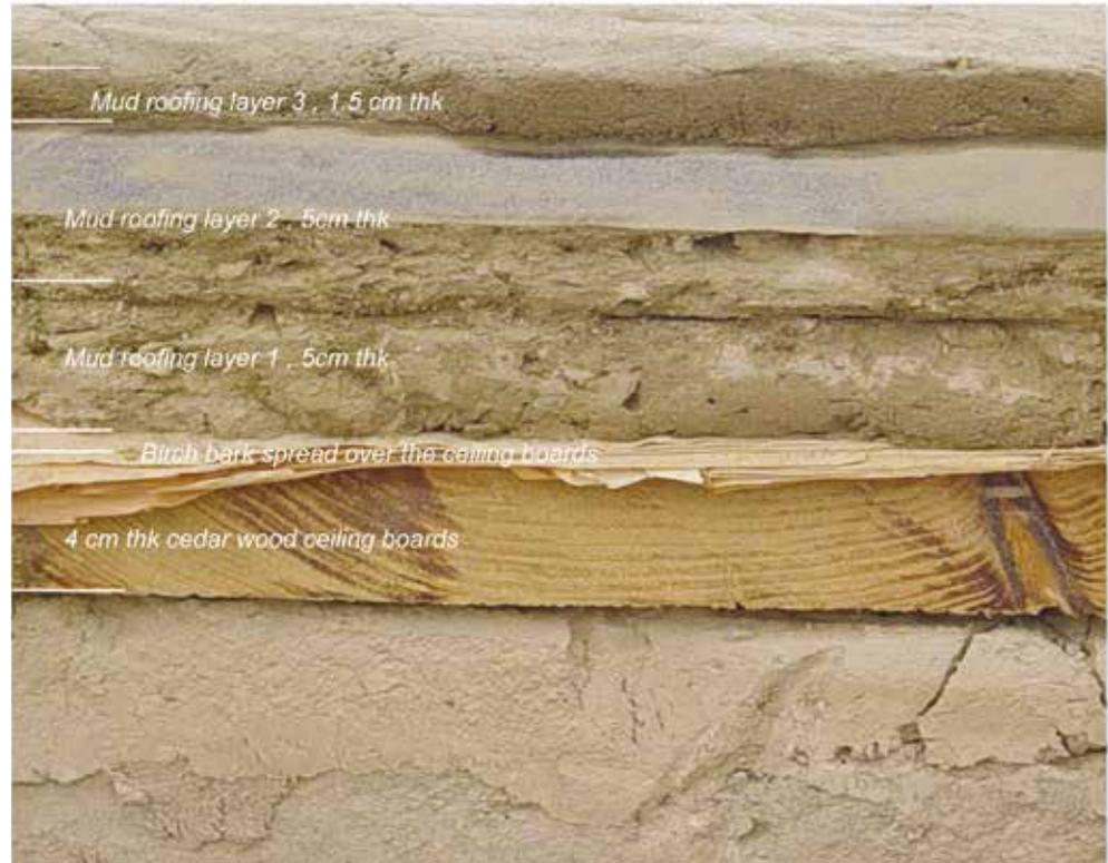
Fig. 182: Restored roof of Lhakhang Gongma. Layers of protection using traditional techniques.
