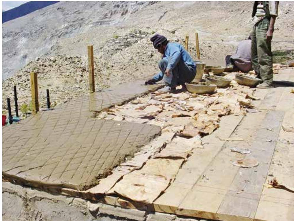
Fig. 58: Flat compacted mud roof being reconstructed at Nako.
