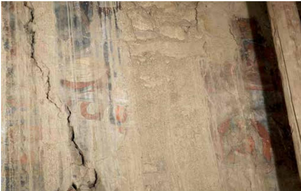
Fig. 242: Cracks and drips with clay deposits, apse in Lotsawa Lhakhang.
