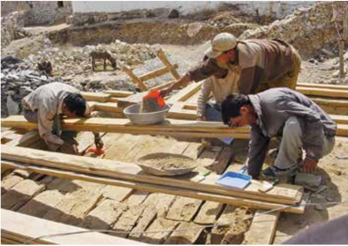
Fig. 188: Careful removal of the thick earth layer on the roof of Lhakhang Gongma.
